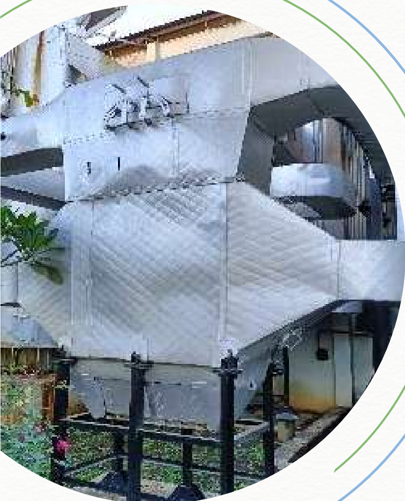
Recuperator to recover heat from flue gas to heat incoming air in ETB
